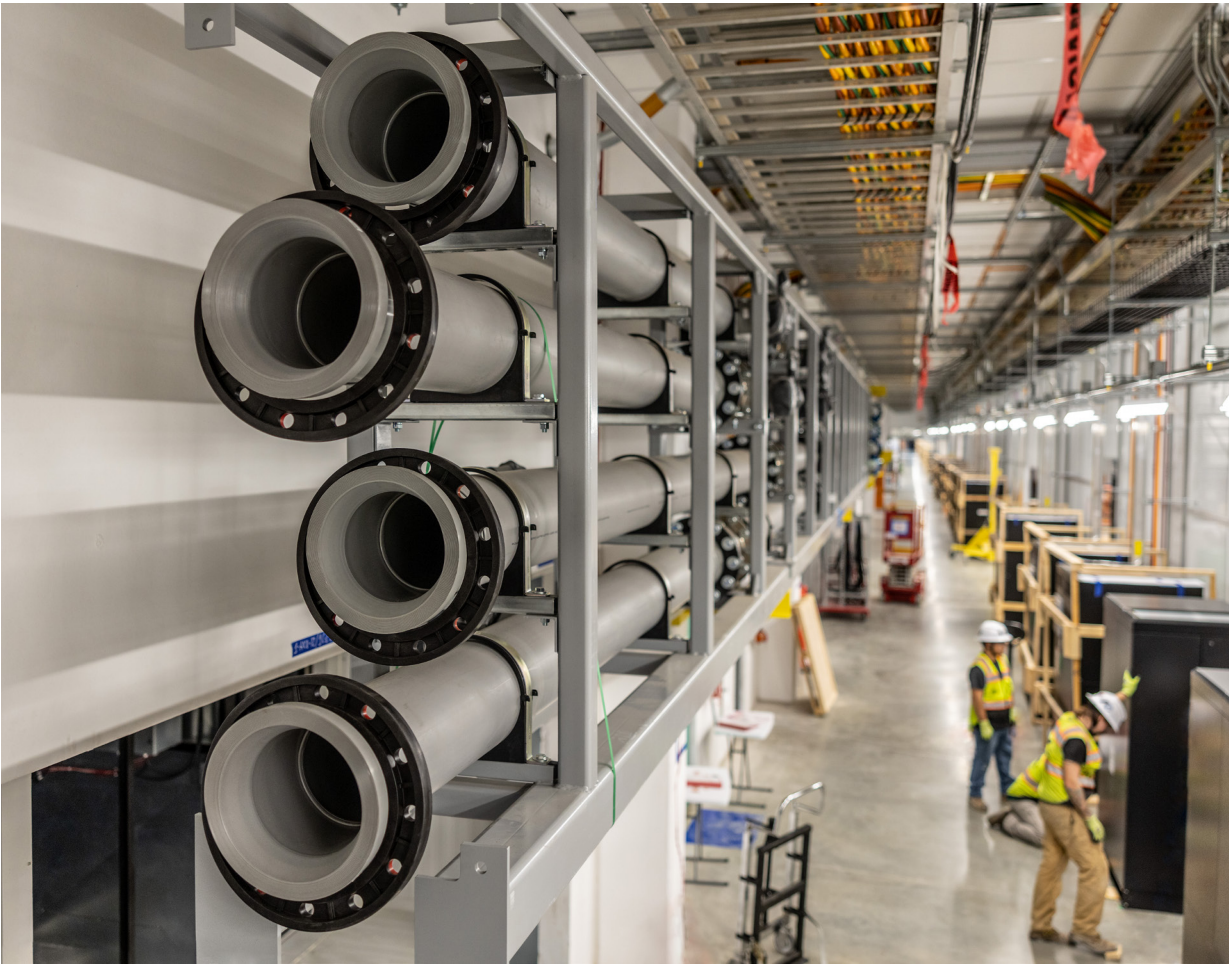
Photo: RK and Compass collaborated to create two innovative first-of-kind fabricated piping systems: the FWS and TCS pipe racks.
